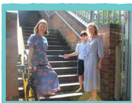
9 year old Jacob asked me for this cycle rail. I was delighted to work with Network Rail to install it.
